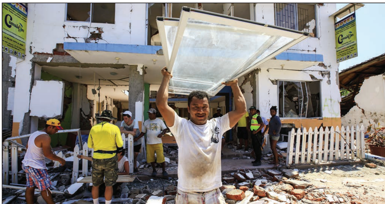
Residents recover some of their belongings on April 25 from debris of a destroyed building in Canoa, Ecuador. Catholic agencies will begin building temporary shelters for thousands of families displaced by the April 16 magnitude-7.8 earthquake, the country's worst natural disaster in nearly seven decades. (CNS photo/Jose Jacome, EPA, Reuters)
