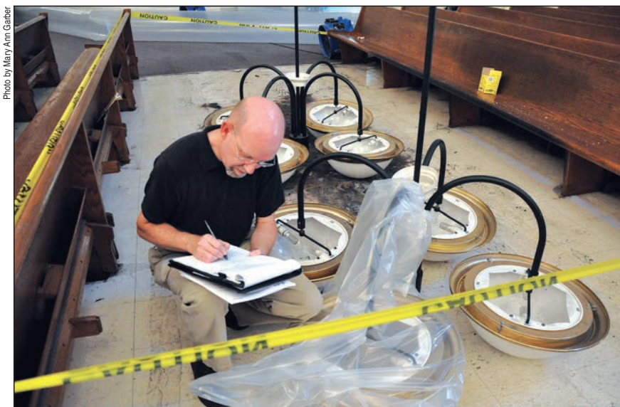
Eric Atkins, director of management services for the archdiocese, inspects the light bulb and chandelier that caused a fire on June 2 at St. Christopher Church in Indianapolis. No estimate of the fire, smoke and water damage is available yet. Restoration work began shortly after firefighters extinguished the blaze.
