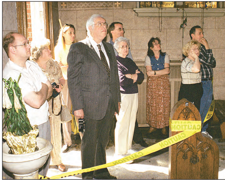
Above: Parishioners survey the damage from the fire, cringing at the destruction of the high altar and the extensive water and smoke damage. Also destroyed in the blaze were stained-glass windows and statues that are irreplaceable.
