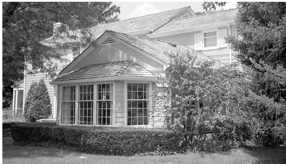
#1 Grade Red Cedar Shingle with Copper Flashing
